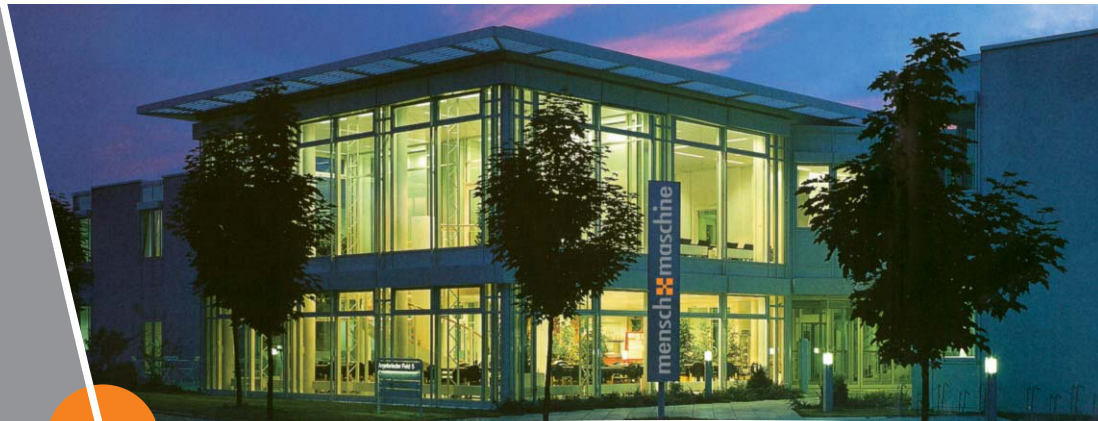
The M+M headquarters in Wessling near Munich
